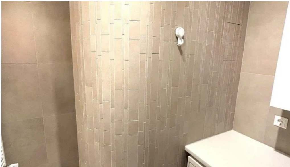
Mr fixer renovations repairs badezimmer
