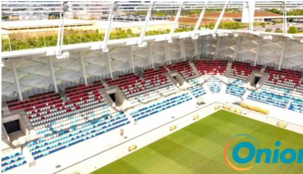
Karp kneip constructions innenansichten
