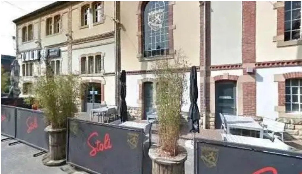
Tero river house luxembourg street view 360deg fotos
