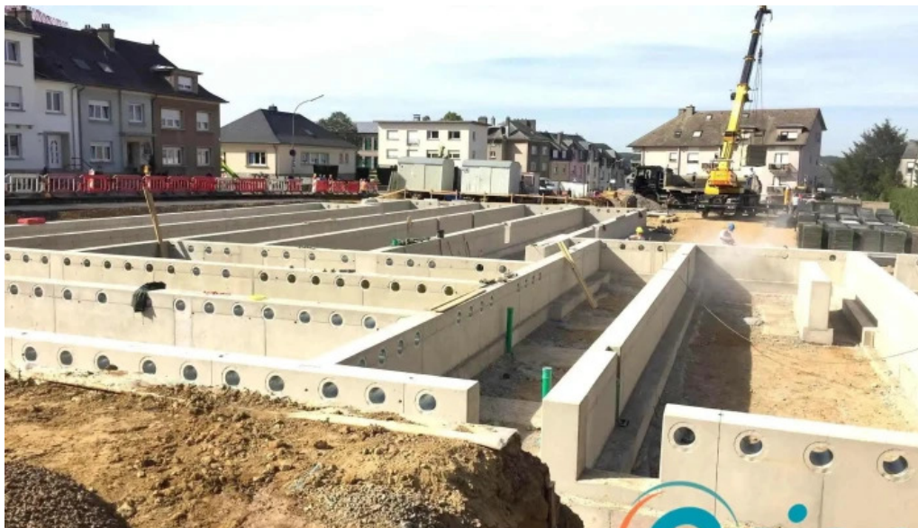
Dz construct telefone
