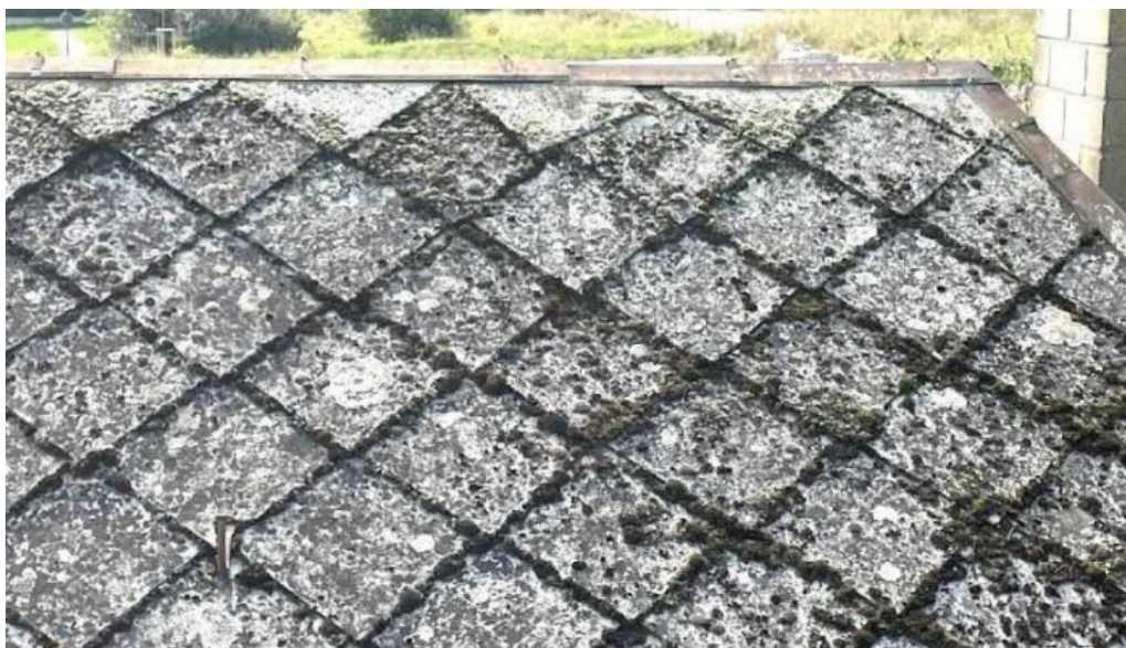
Renov hous kaerjeng
