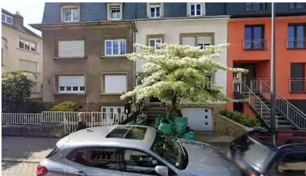
Net clean sarl street view 360deg fotos
