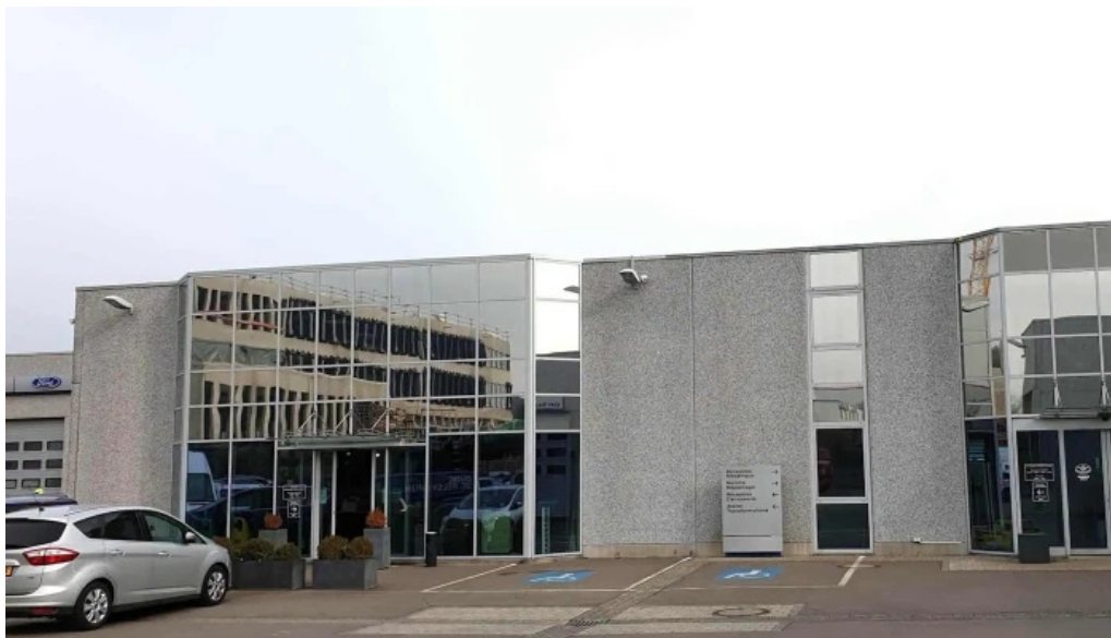
Fordstore autopolis niederkorn differdingen
