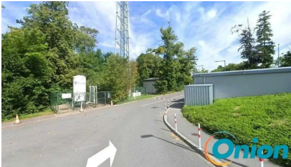
Chargy charging station bad mondorf
