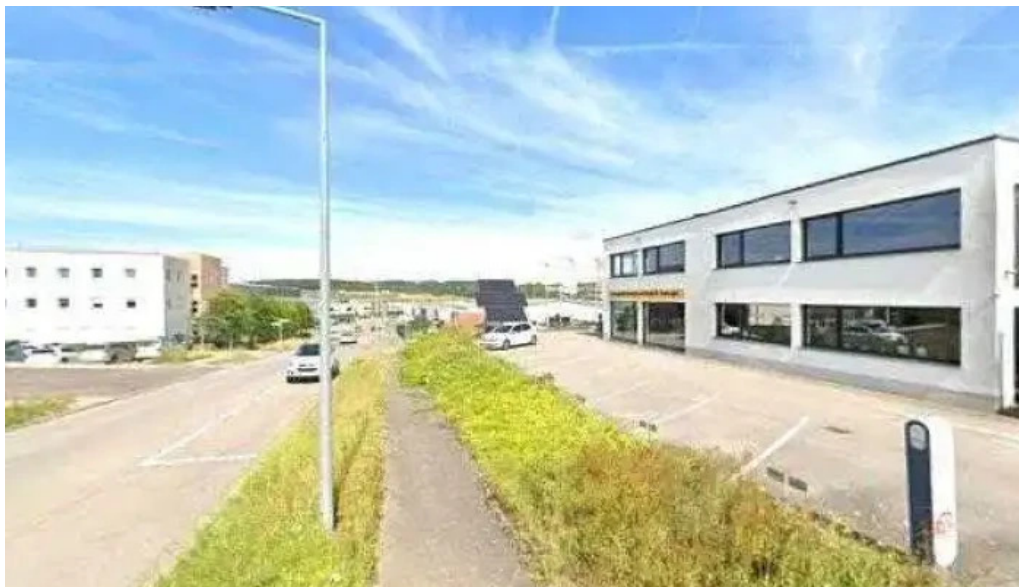
Enovos charging station locatione
