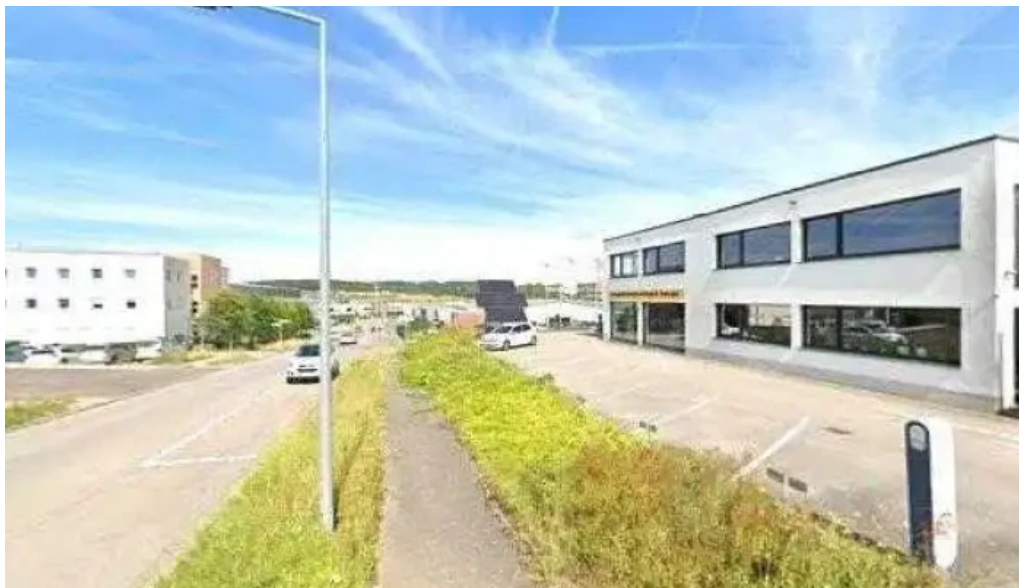
Enovos charging station street view 360deg fotos
