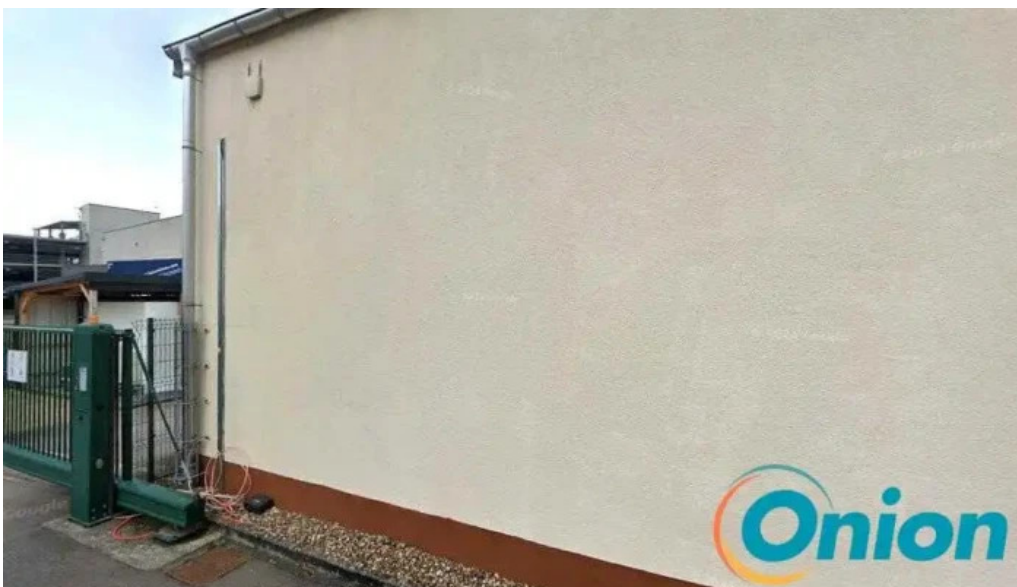
Chargy charging station biwer
