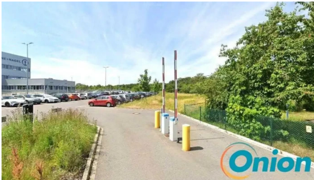
Totalenergies charging station contern
