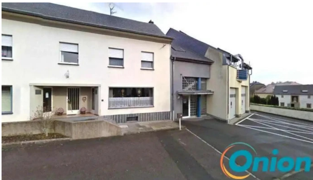
Administration communale de garnich cultural centre charging station garnich
