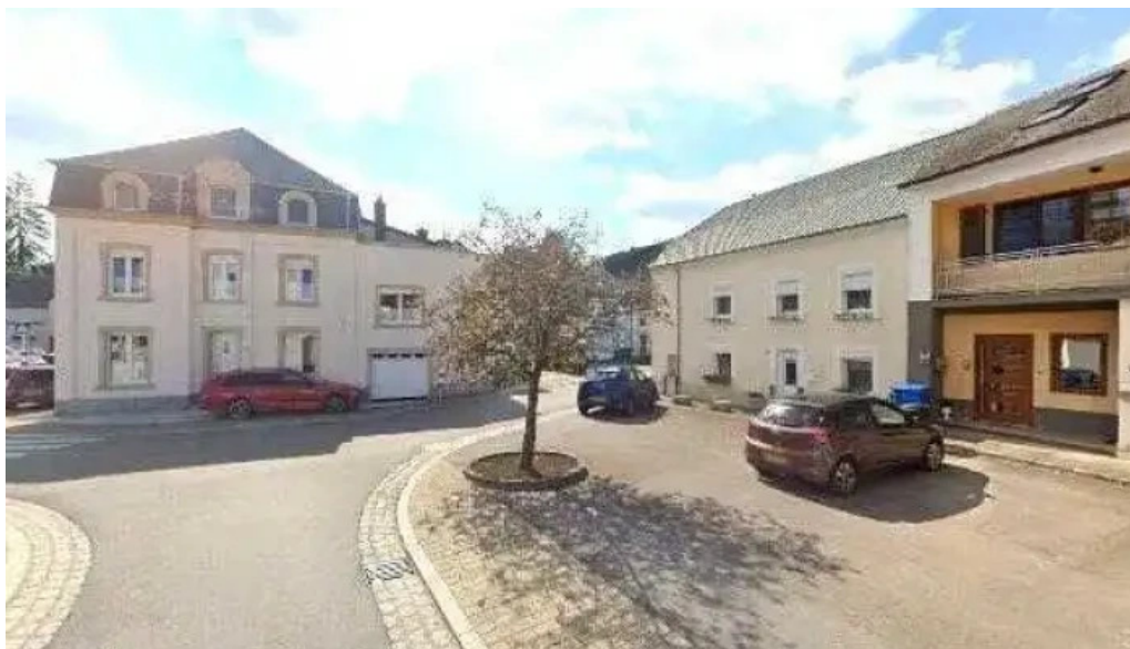
Chargy charging station adresse
