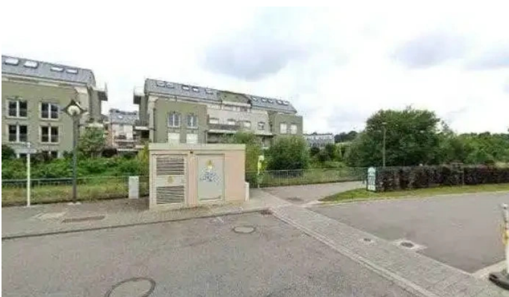
Chargy charging station woue
