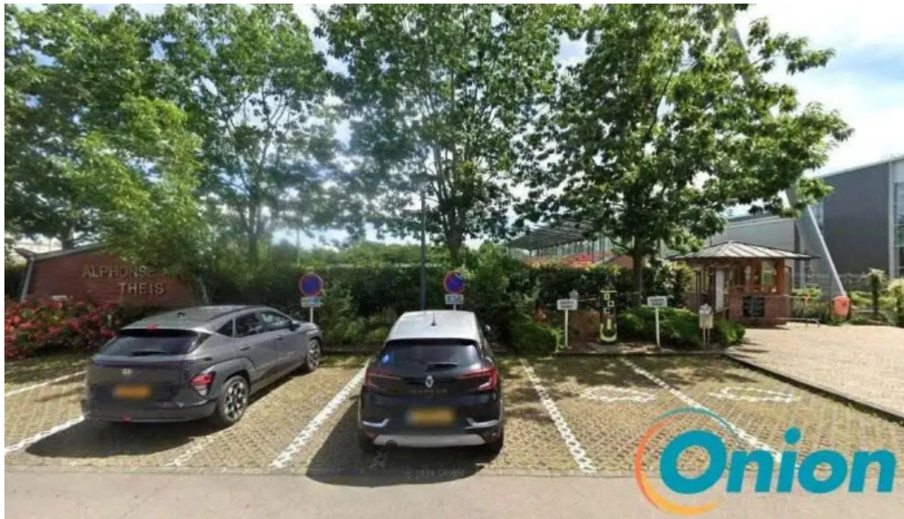
Chary charging station hesperingen
