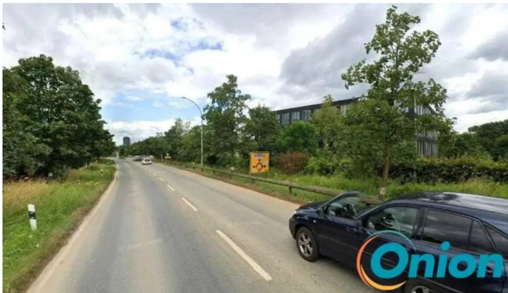
Electric vehicle charging station hesperingen
