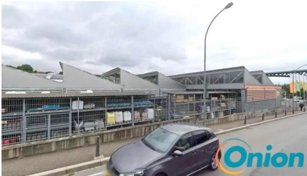
Enovos charging station junglinster
