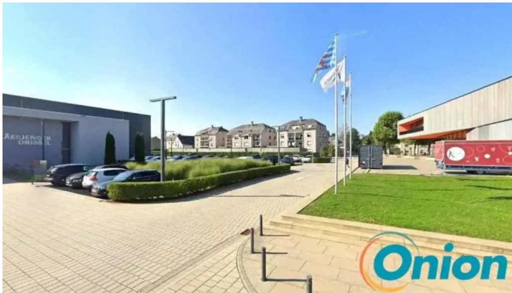
Chargy charging station kaerjeng
