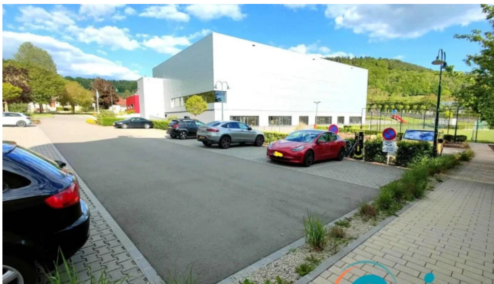
Chargy charging station praissere
