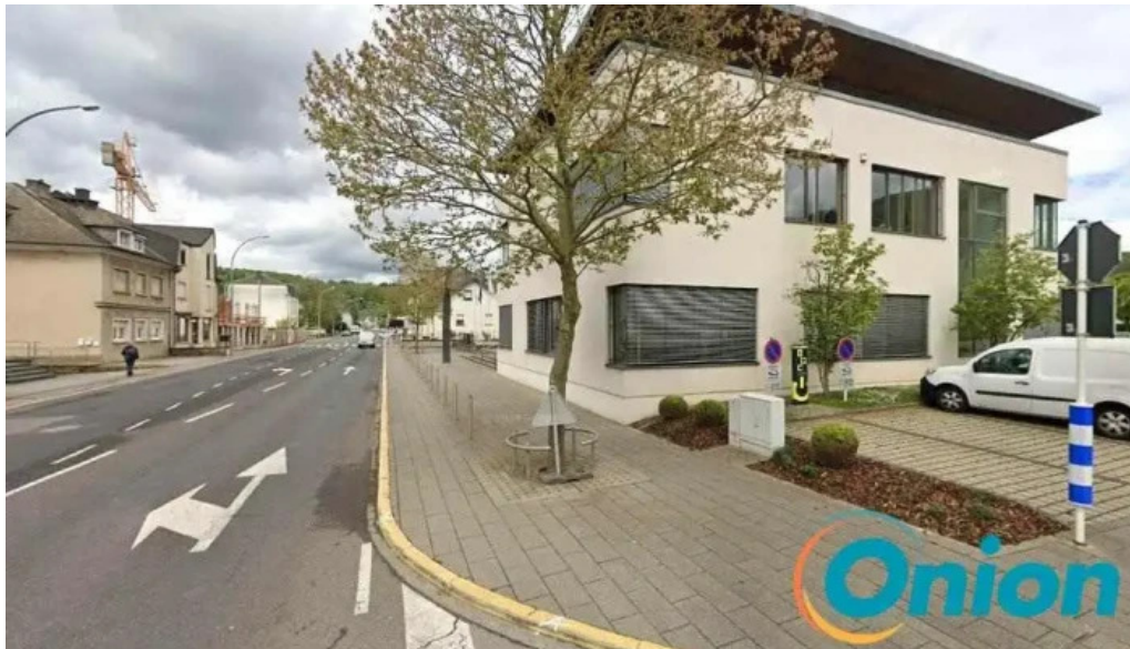
Charge charging station lorentzweiler
