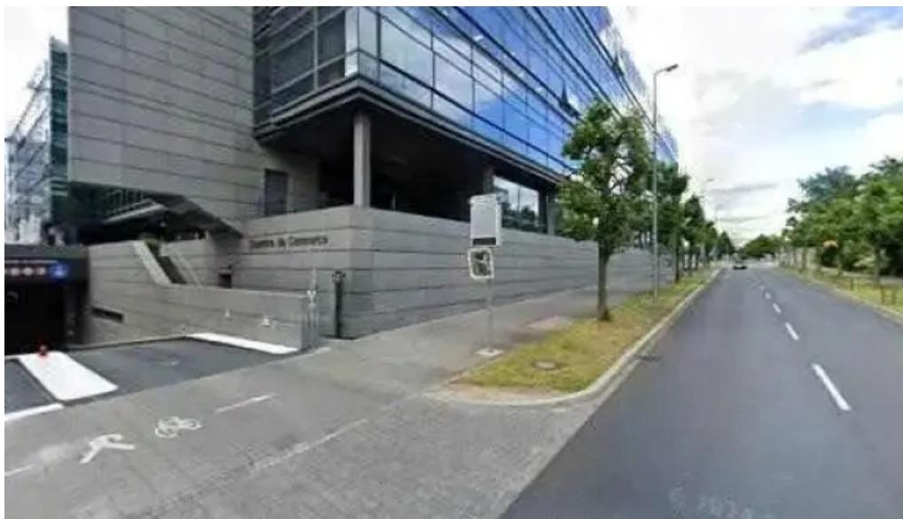
Chargy charging station locatione
