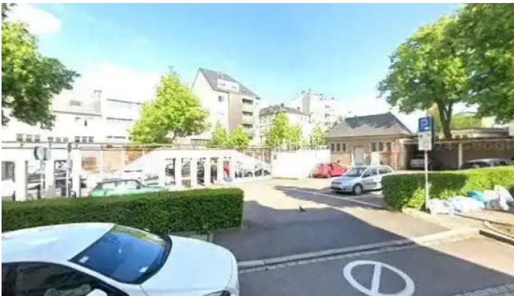
Chargy charging station woue
