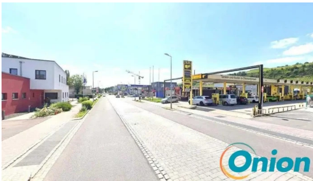
Chargy charging station mertert
