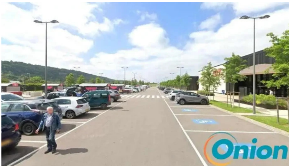
Pc tank s a r l ladestation mertert
