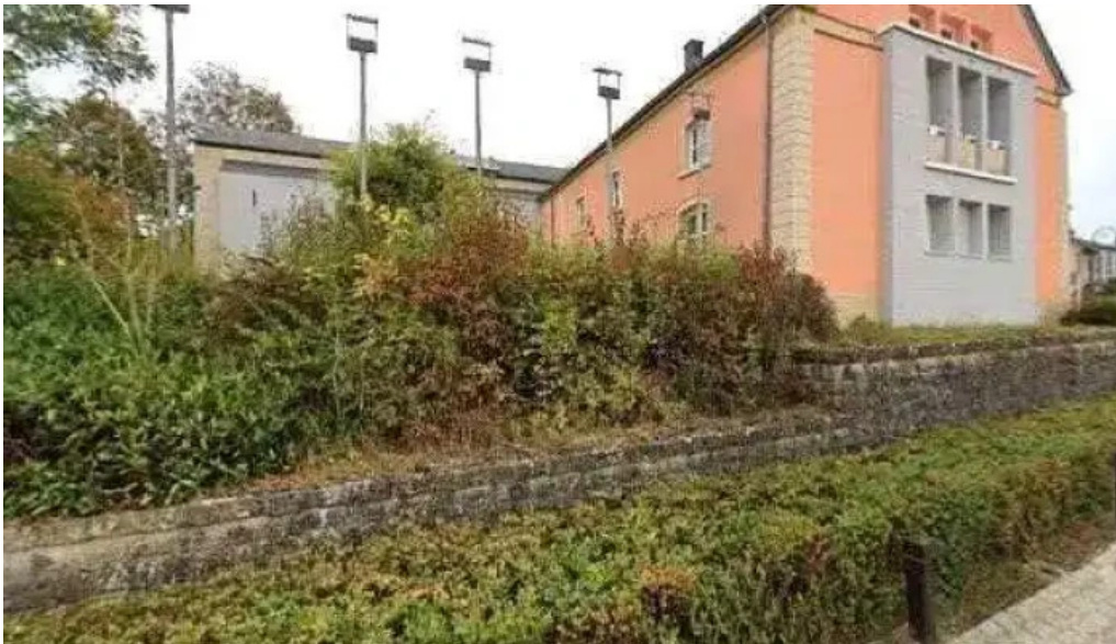
Chargy charging station remisene
