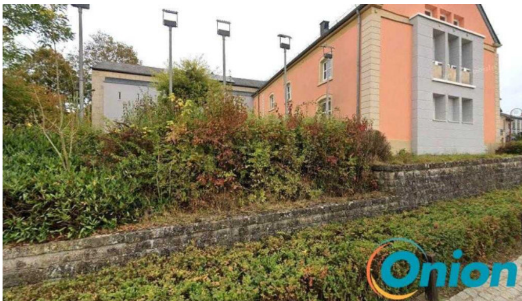
Chargy charging station reckingen mess
