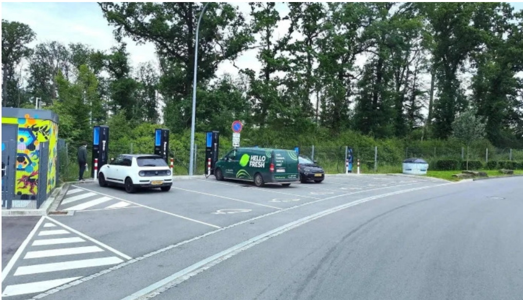
Superchargy ladestation bewaertung
