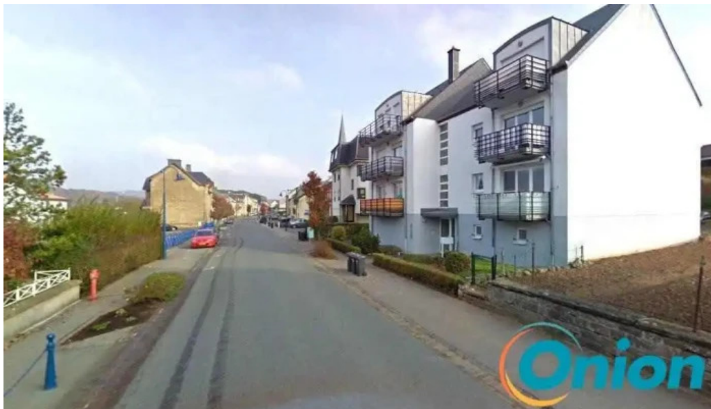
Chargy charging station schieren
