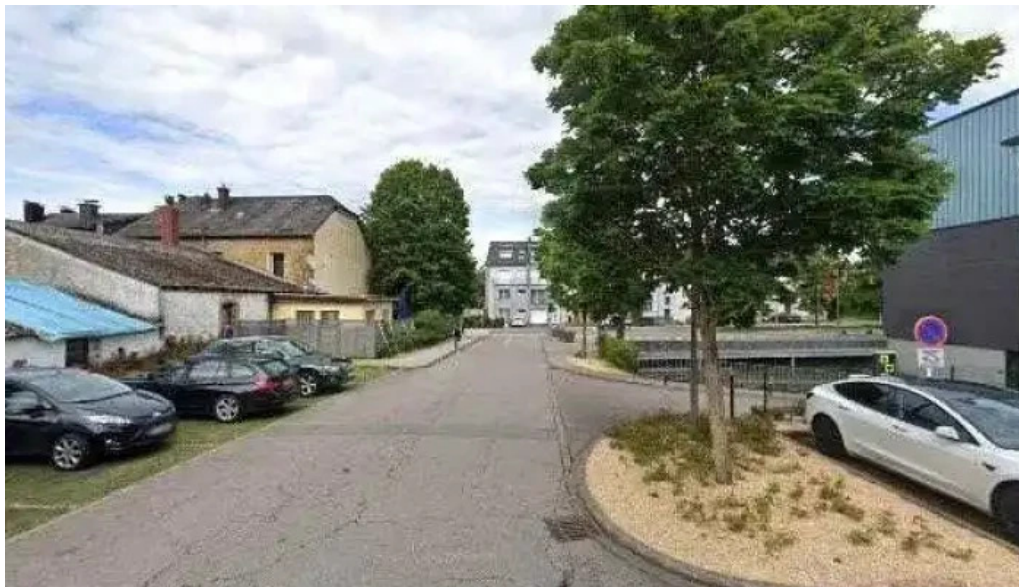
Chargy charging station stonnenplange
