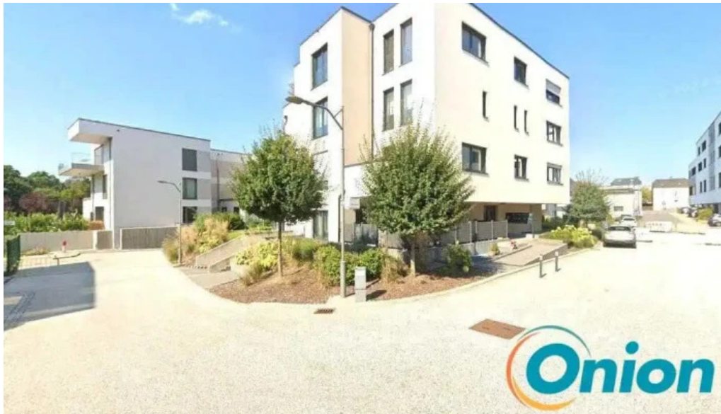
Chargey charging station steinfort
