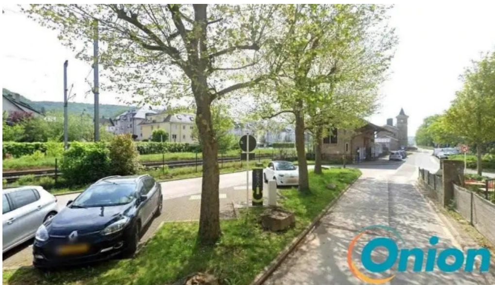
Chargy charging station strassen
