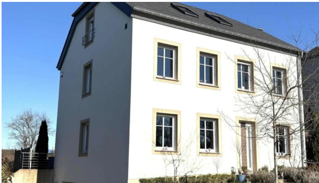
Taff sa rl by wandwerk befort
