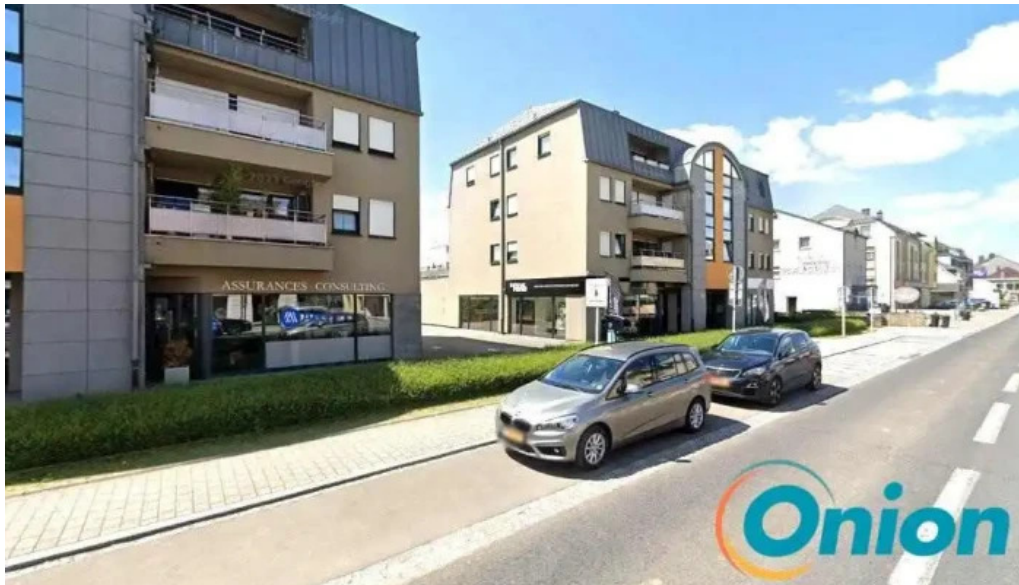
Bini electricite maintenance strassen
