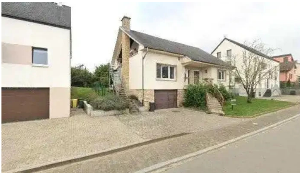
Mp construction remisene
